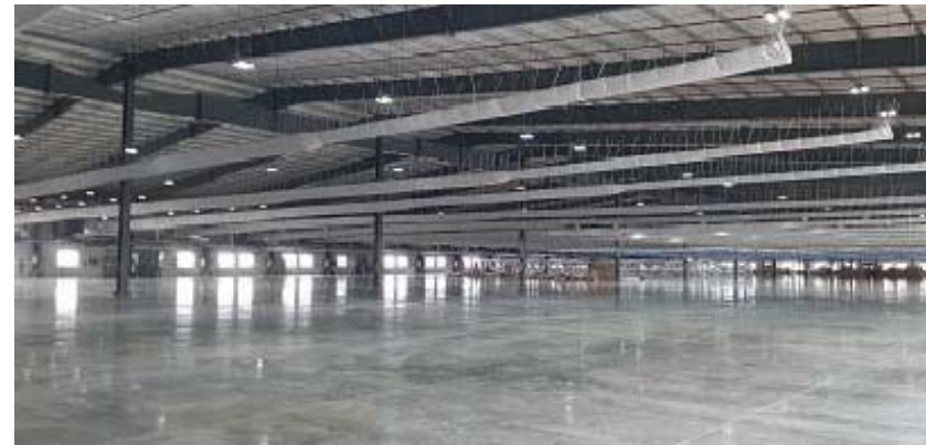
Main Bldg Flooring & PEB
