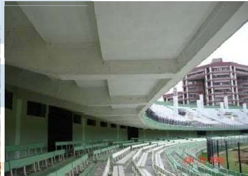
Finished stands of tier 1 after completion
