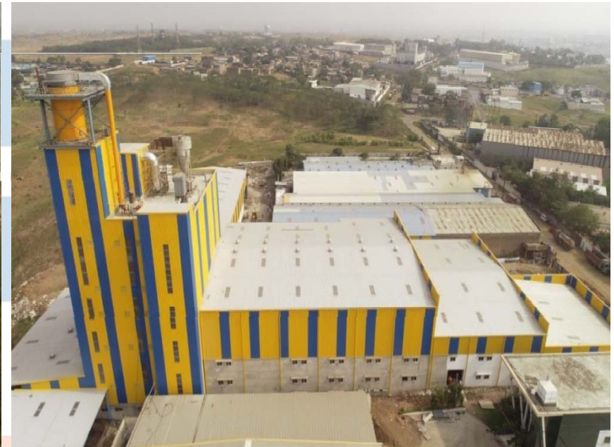
Side view of 54 mtr high Pre-Engineered Process Tower
